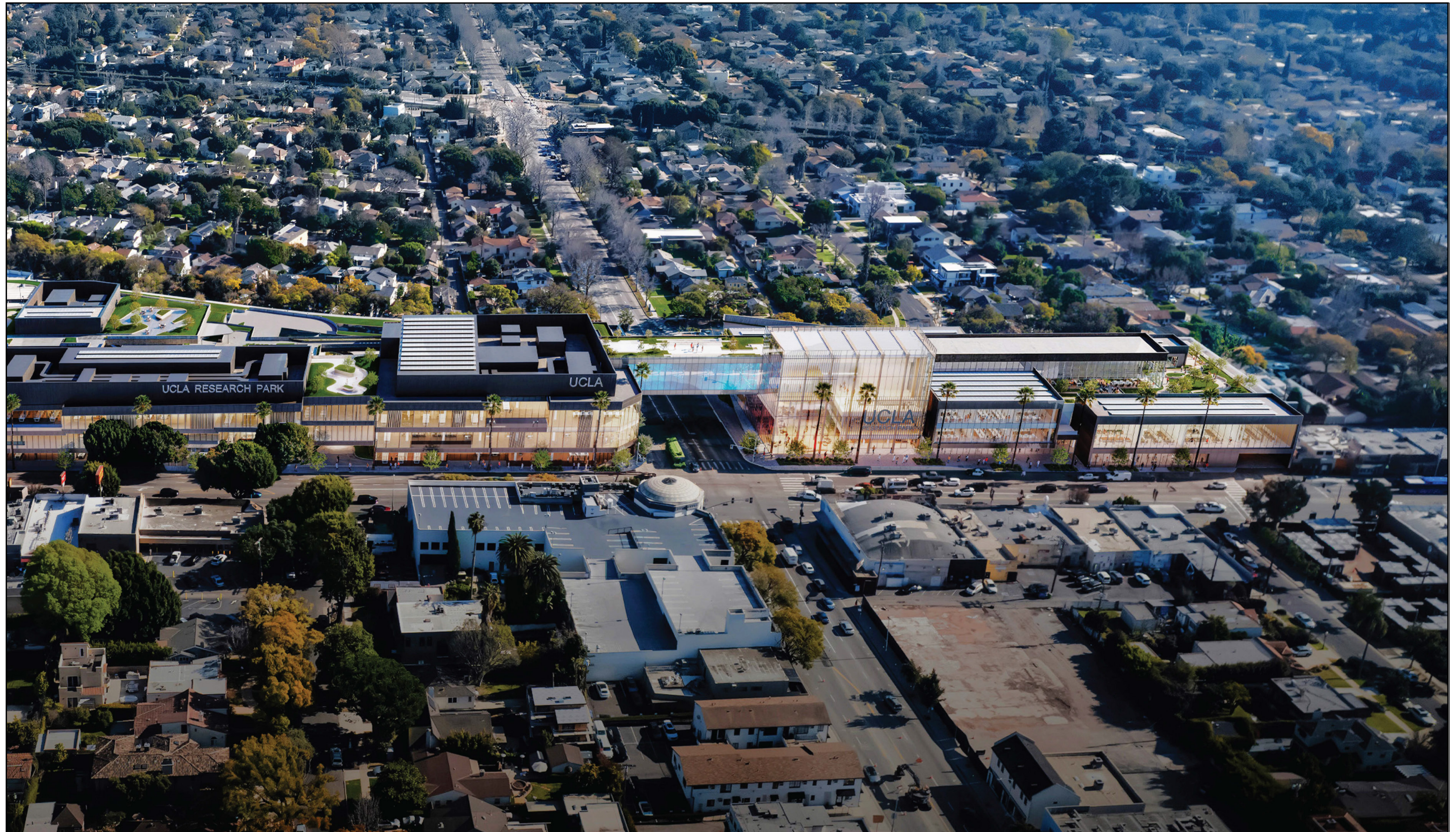
Source(s): Flad Architects (2026)
