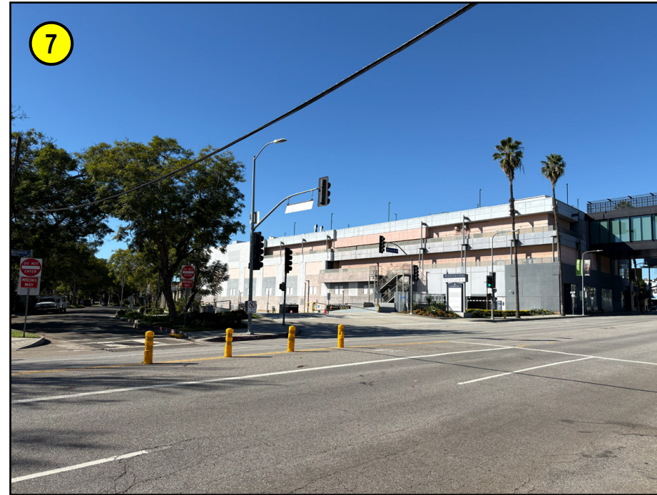
Site Photo 7: South of the Project Site at the intersection of Aryes Avenue and Westwood Boulevard looking northwest.
